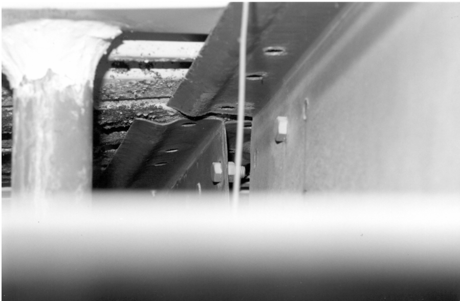
Figure (5) Relative movement of floor at the line above the middle girder.
