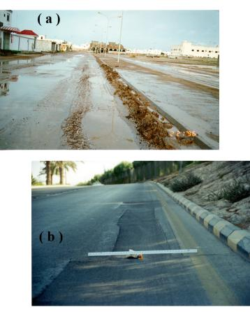
Figure 1. Typical road deterioration in the Dammam area (a) due to the use of water sensitive calcareous sediments as a graded base layer and (b) due to poor construction of utility trenches
